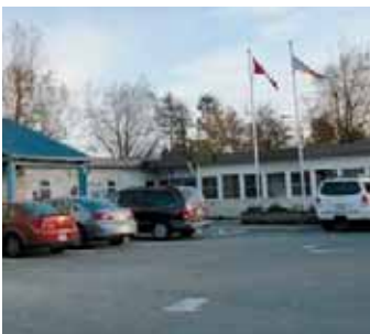
SOUTH POPLAR ELEMENTARY
